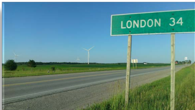
Adelaide-Metcalfe wind energy development, Ontario
